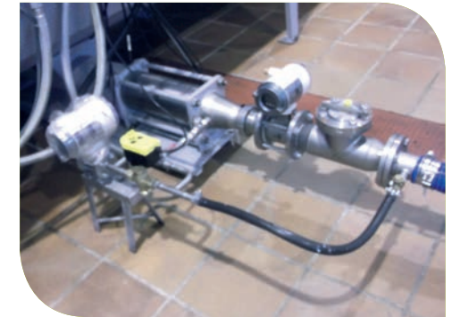
Picture 1: Humidity sensor installed in the entrance of the decanter.
